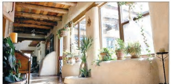
About 100 hand-peeled vigas can be found in the home. In addition to being load bearing, the vigas complement the tongue-and-groove ceiling.
